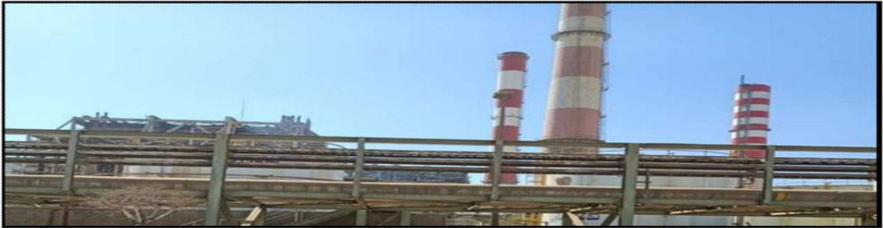
Assiut thermal power plant (units I,II (2*300MW) and unit III (1*650) ) Image (3)
